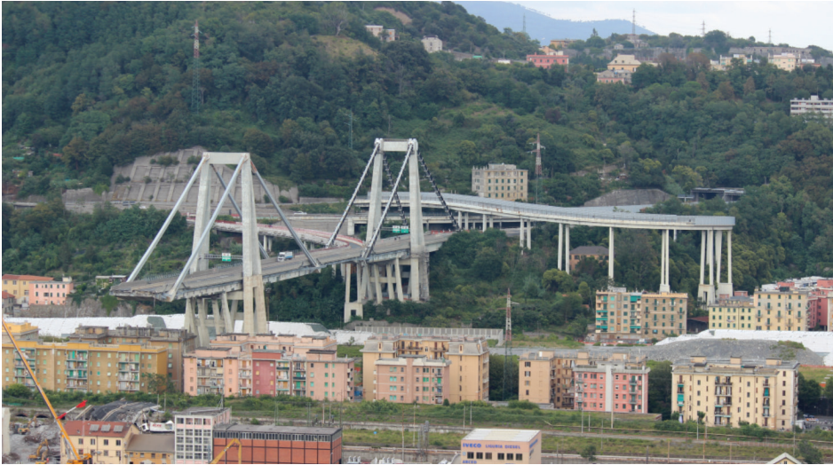
Photo of the Ponte Morandi taken on August 25, 2018, nine days after its collapse.
