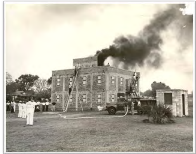
Burn building at original campus
