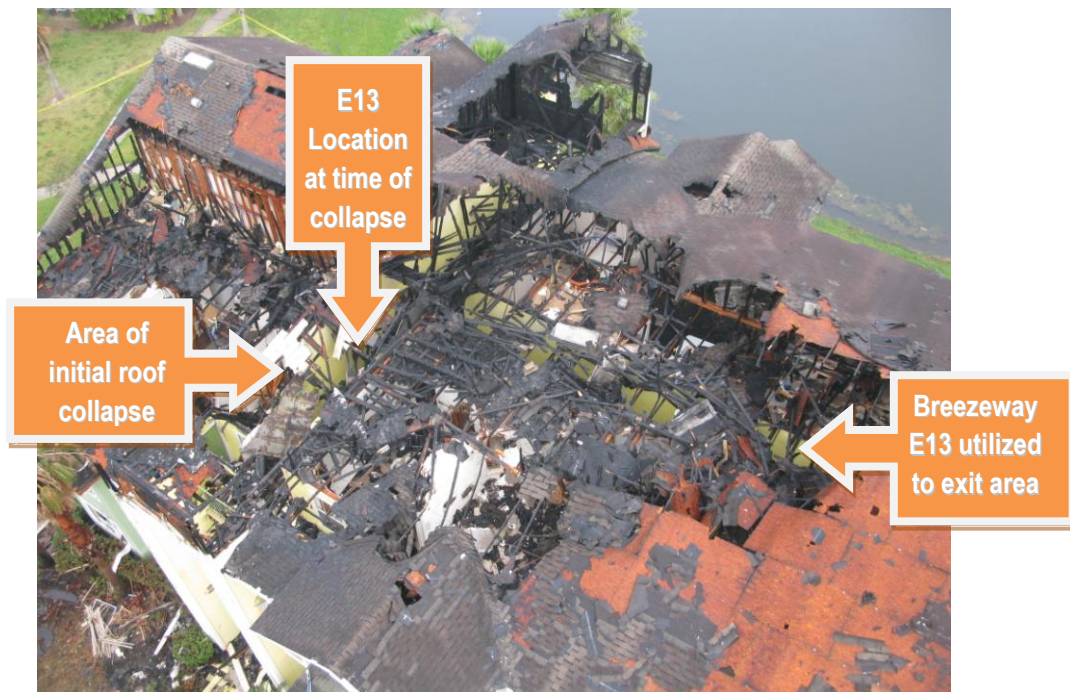
Picture 5 – Aerial view of 3 rd floor Side B stairwell landing & breezeway.
