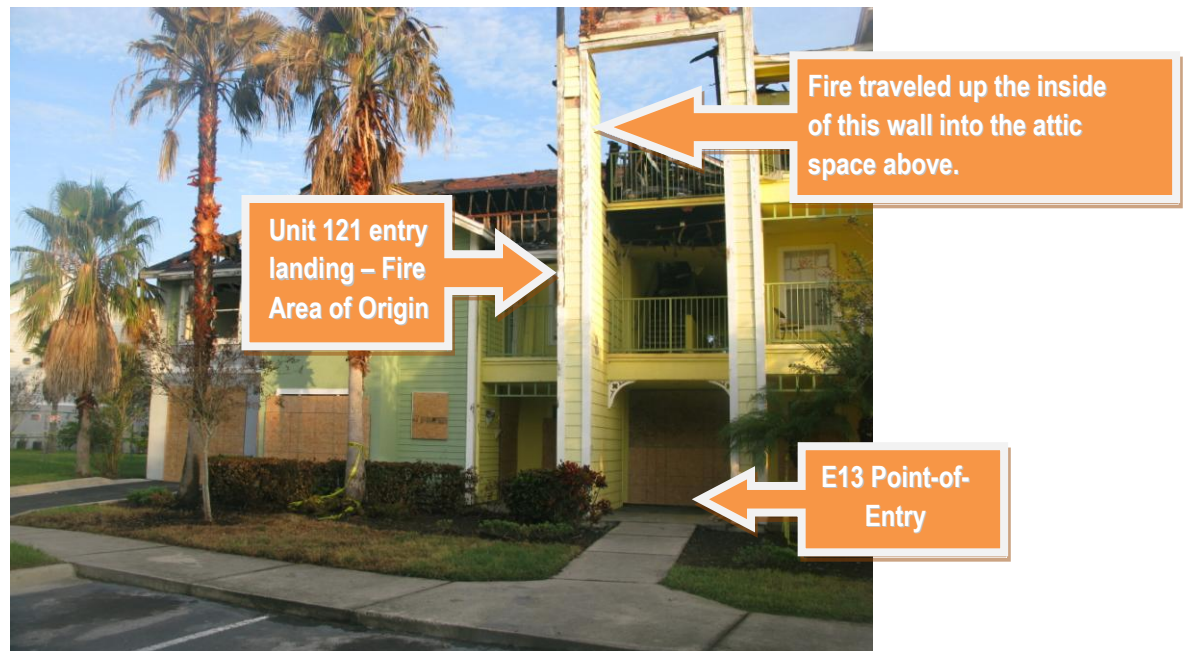
Picture 3 – Side A at E13's point-of-entry to B Side stairwell.
