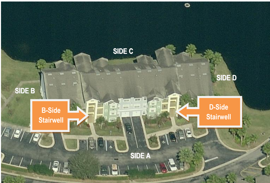
Picture 2 – Northward view of 4103 Tropical Isle Blvd noting Side B and Side D stairwells.
